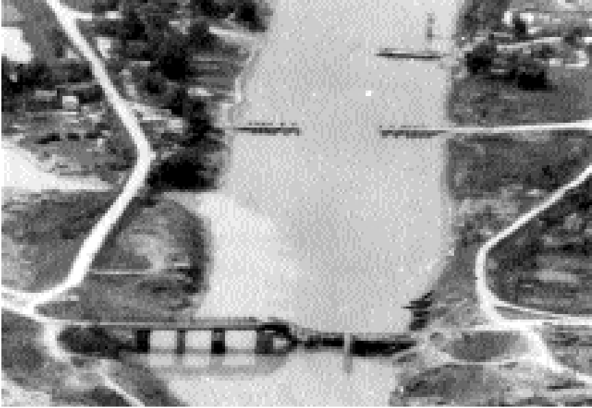
Bac Giang bridge after the May 5 attack. A pontoon bridge and a ferry are above the destroyed bridge.
