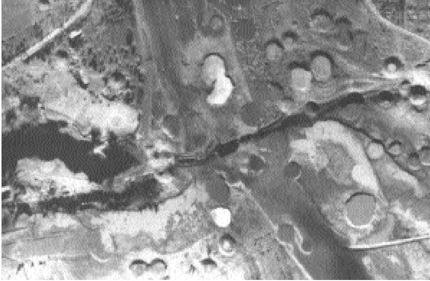
The Bac Can highway bridge, located about seventy-five miles north of Hanoi, after an F-105 strike in December 1965.
