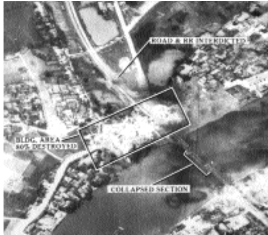
Dong Phuong Thuong railroad and highway bridge after attack.
