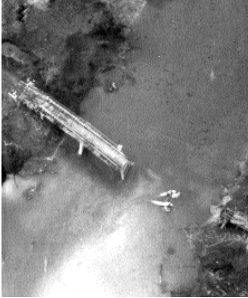
The Lang Met highway bridge on Route 1A north of Hanoi, October 1965.
