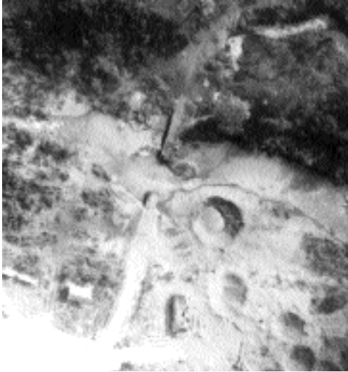
Kim Cuong highway bridge after attack.
