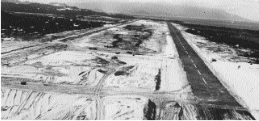
Runway construction at Cam Ranh Bay.
