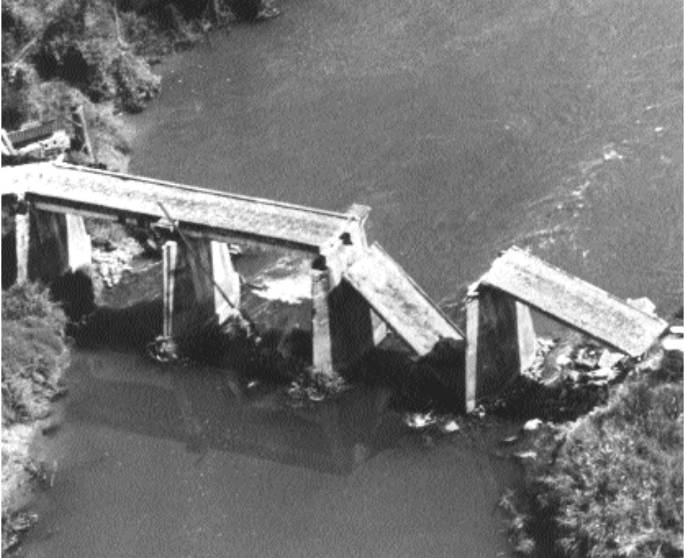
Bridge damaged by bombing in 1965.
