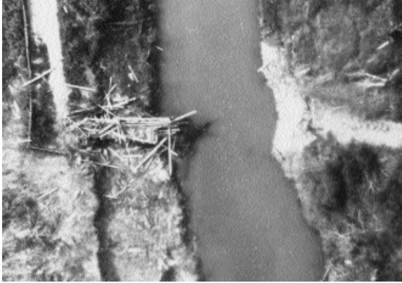
Bridge on Route 6 southeast of Dien Bien Phu destroyed by Air Force F-105s.
