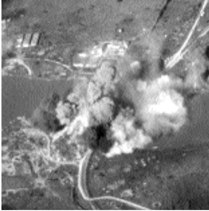
Thanh Hoa highway and railroad bridge under attack.
