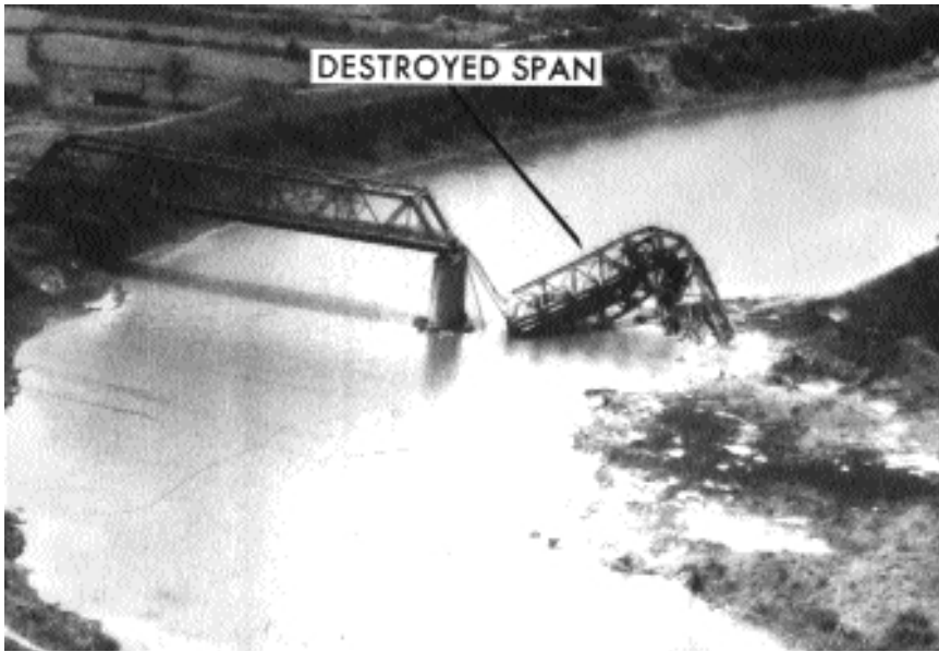
Qui Vinh railroad bridge after an attack in April 1965.
