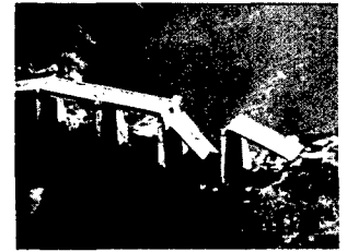
Destroyed bridge in Laos, 1965.
