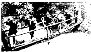
Viet Cong troops cross an improvised foot bridge in South Vietnam.
