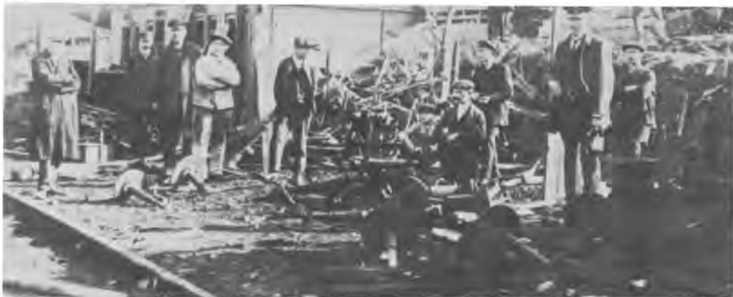
Damage to a railway station near Luxembourg.
