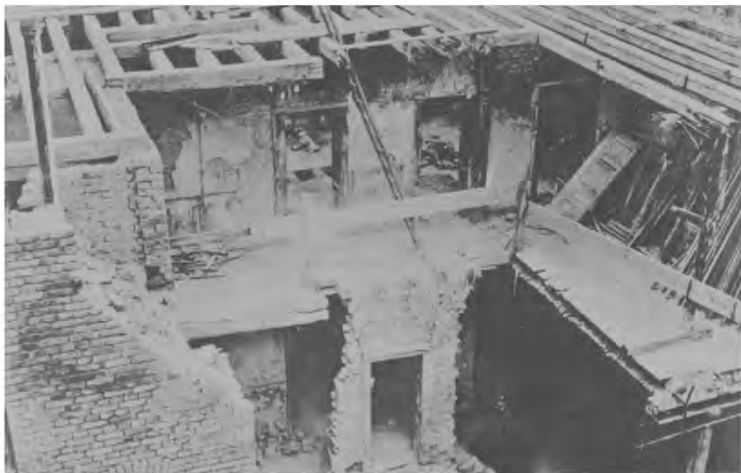
Damage caused by a 1,600-lb. British bomb.
