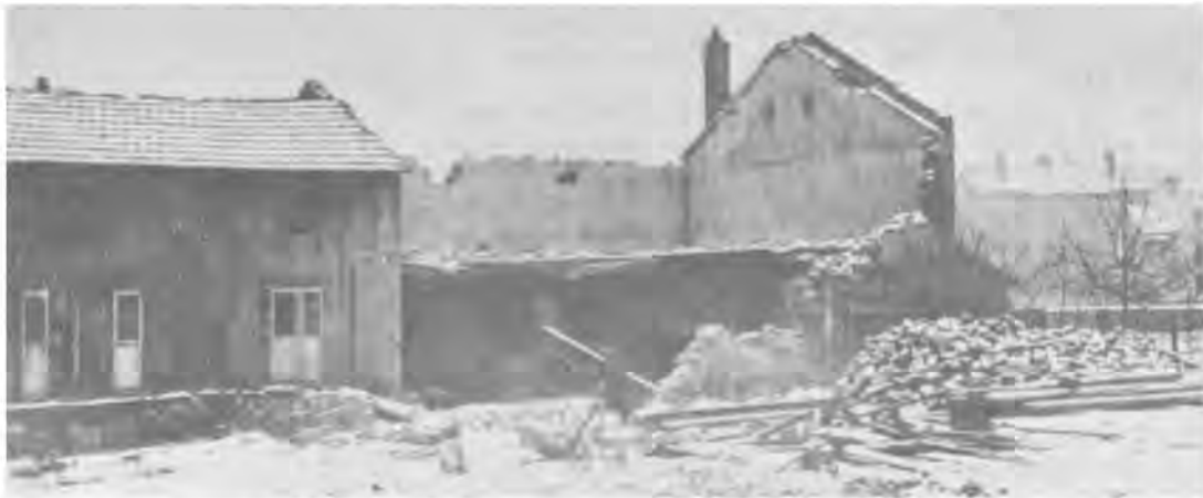
The explosion of a 112-lb. British bomb collapsed the wall of the building in the photo.
