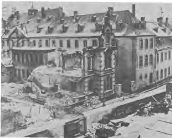
The damage above, caused by a 230-lb. British bomb, was termed "considerable" by World War I assessments.
