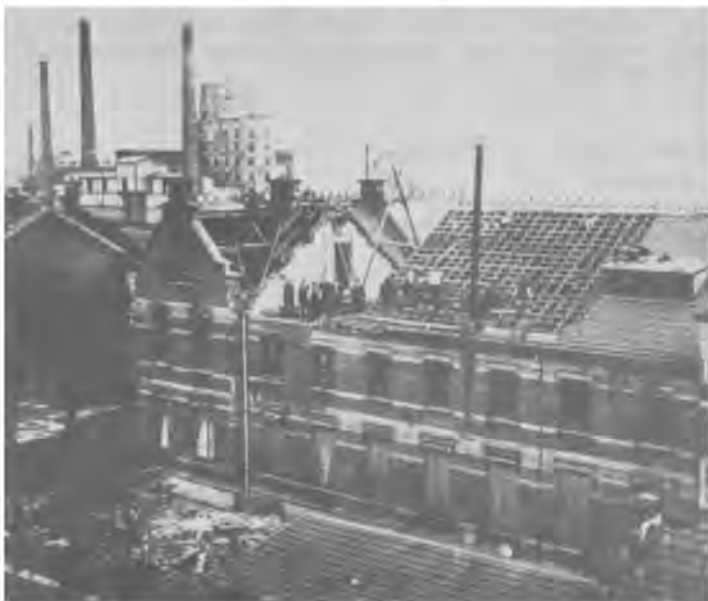
Office of the Solvay Chemical Factory at Sarralbe, following the air raid of 22 August 1918.
