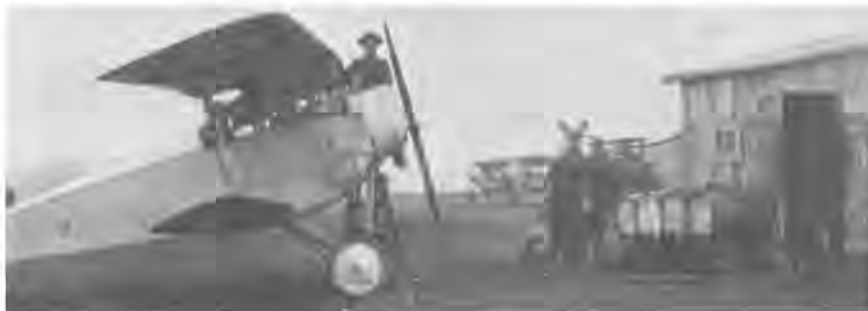
Gas and oil refueling station, Issoudun.
