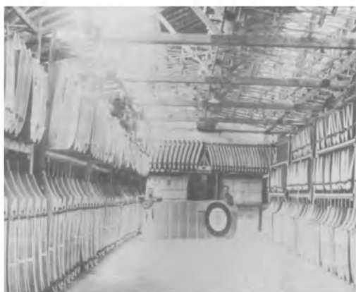
Wing room of the Aero Supply Depot, AIC, Issoudun.
