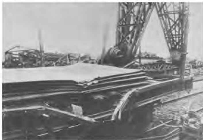
Damage at Volklingen.
