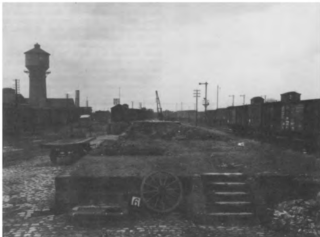
Thionville railroad station.
